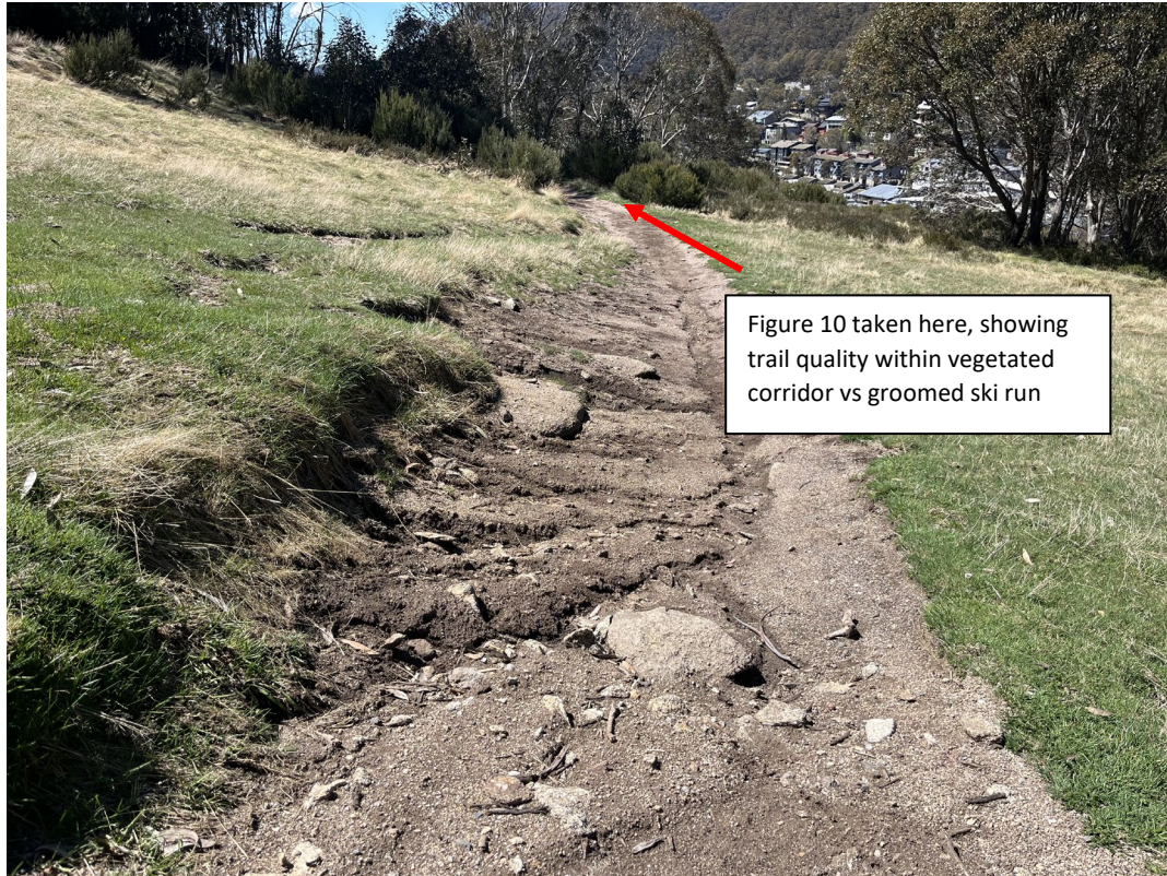
Figure 9: Evidence of trail erosion on groomed Milk Run ski run. Photo taken October 2023.
